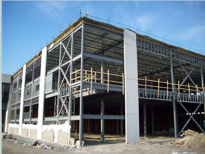
Polyval's new warehouse under construction
